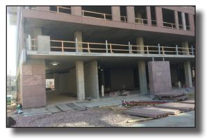
The exterior panels continue to be installed. We are now adding the stone panels to the west face.
